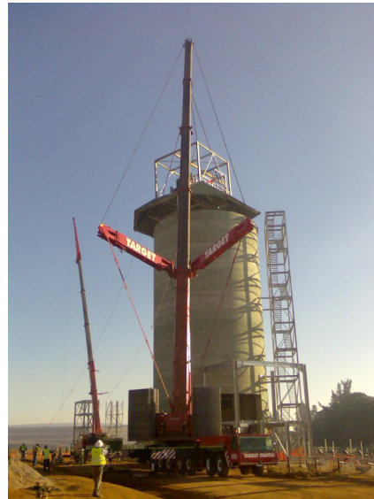
Above: The 440 ton LTM1400 in the process of lifting a trestle.
