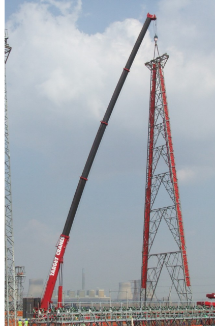
Above: The 440 ton LTM1400 in the process of lifting a trestle.
