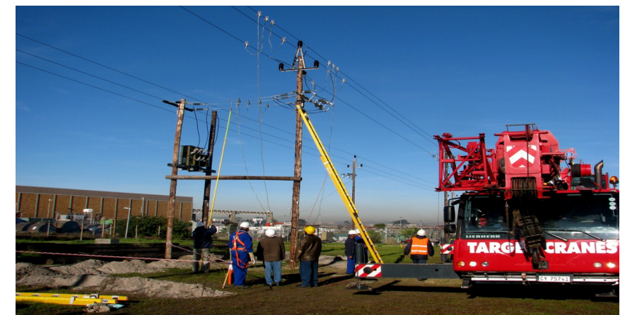
Above: 55ton LTM1060 Liebherr - Eskom in process of earthing connections.
