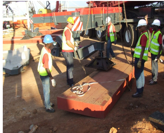
Above: The assemble crew setting up the out rigger pad.
