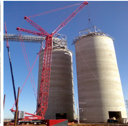
Above: The 600 ton LG1550 lifting the 47 ton silo top structure.
