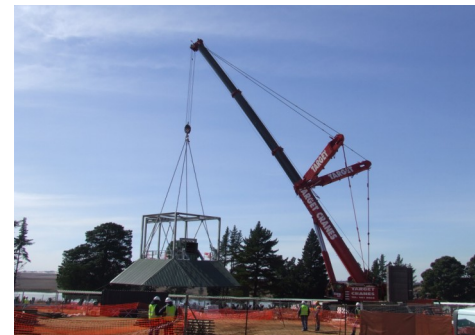
Left: 440 ton LTM1400 lifting 37 ton silo top structure to highs of 37metre.
